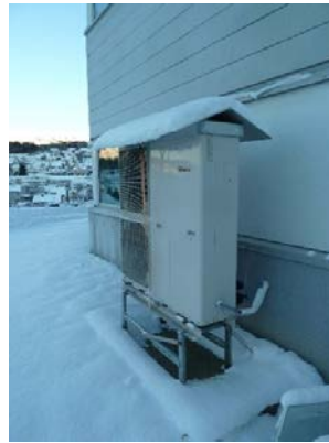
Varmepumpe utedel
